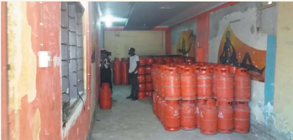
Figure 22: A residential storage area for LPG cylinders with no adequate ventilation
