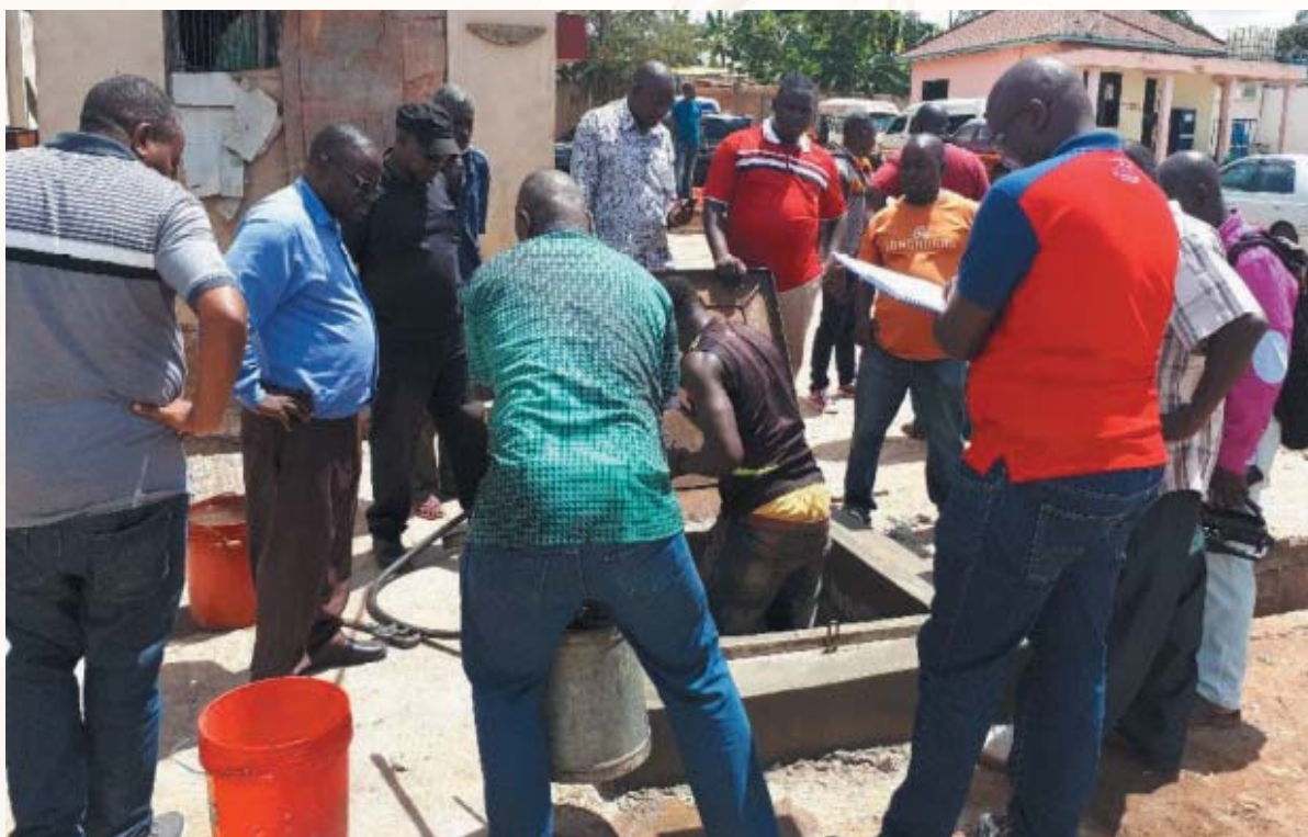
Figure 26: Preparations for Hydrostatic Testing at Buseresere Filling Station
